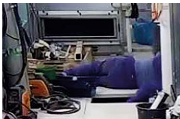
Figure 1: Contractor lying on deck to reach and disconnect mounts
