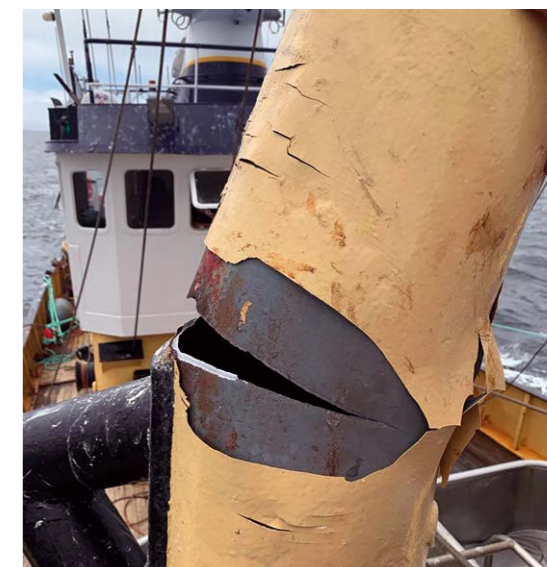
Figure 2: One of the cracks in the derrick posts
