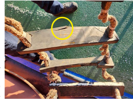
Figure 3: Cracked, warped rubber steps and worn side ropes. The ladder also appears to have been painted
