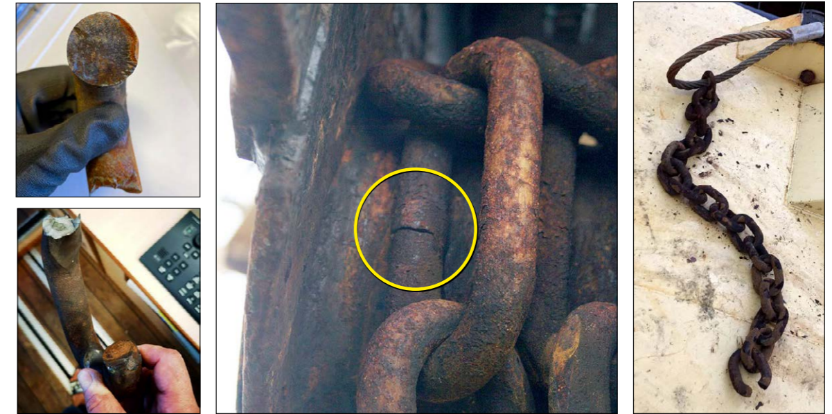
Figure 3: Identified chain defects in static pin arrangements
